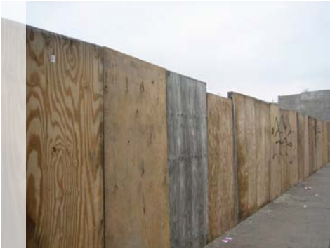
Inactive Frontage: vacant land
